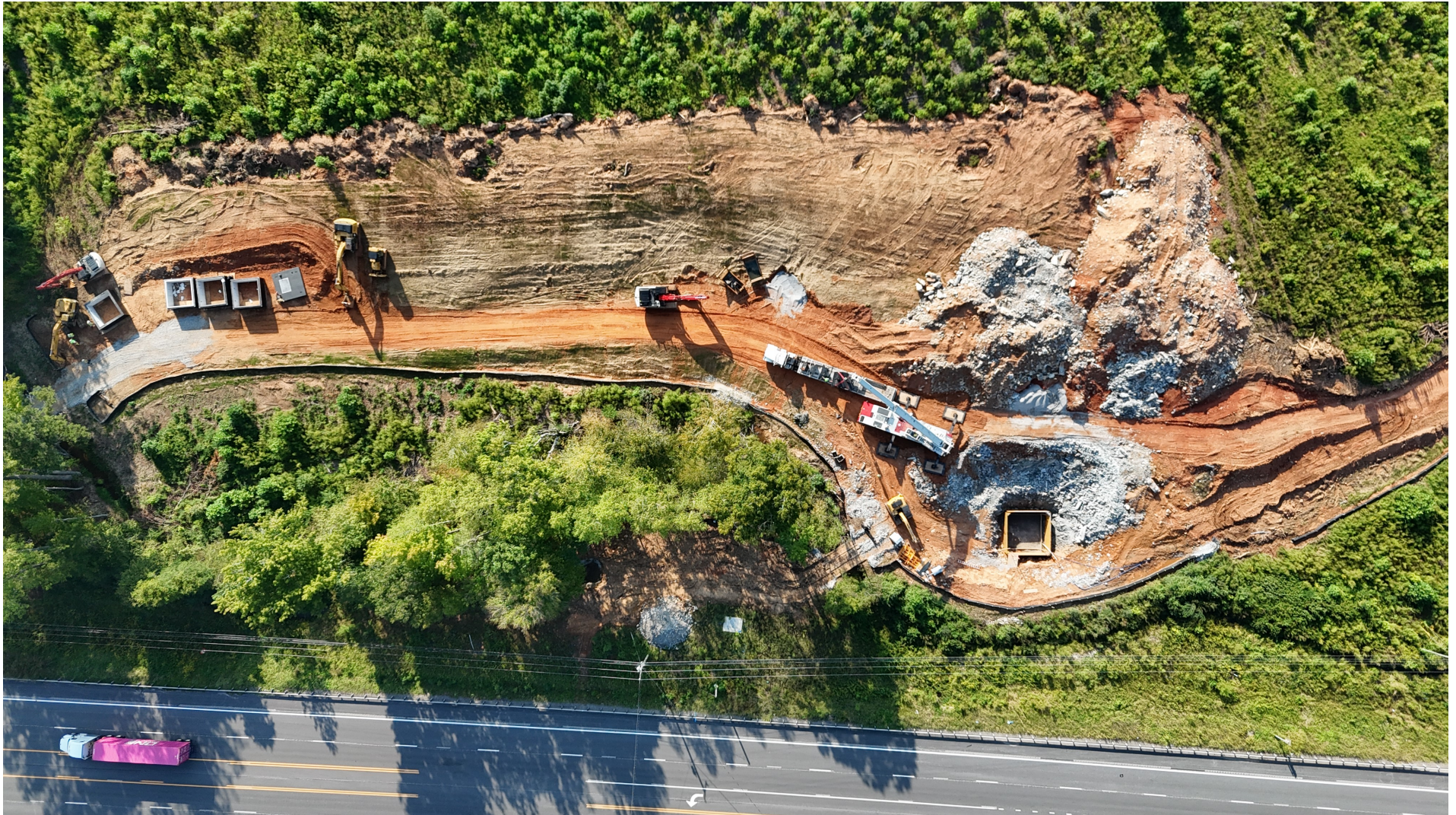
Aerial View looking down on crane setup preparing to stack the pump station. Top left are the five square pump station sections that will be installed using the crane. Crane is sitting next to rock pit. The pump station sections will be installed in the square trench box at the square on the Right side of the picture.
